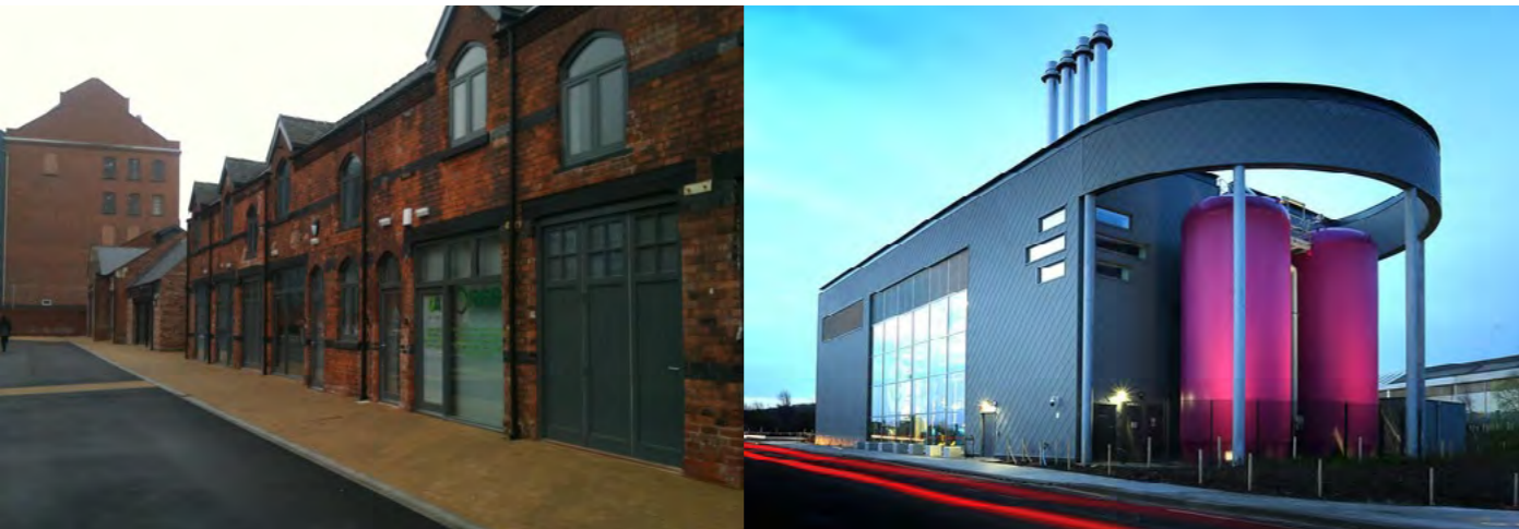
Gateshead Energy Centre.
